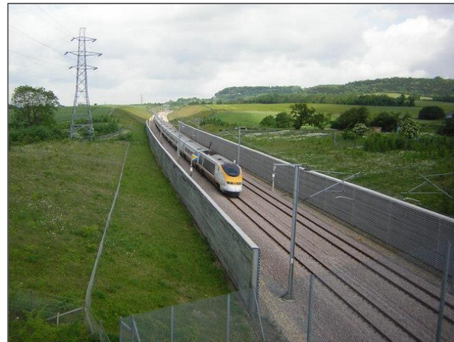
Channel Tunnel Rail Link near Boarley Farm London bound Eurostar speeds along the CTRL near Boarley Farm [obrázek]. Wikipedia: the free encyclopedia . [Cit. 20. 05. 2020] Dostupné z: https://commons.wikimedia.org/wiki/File:Channel_Tunnel_Rail_Link_near_Boarley_Farm_-_geograph.org.uk_-_777007.jpg
